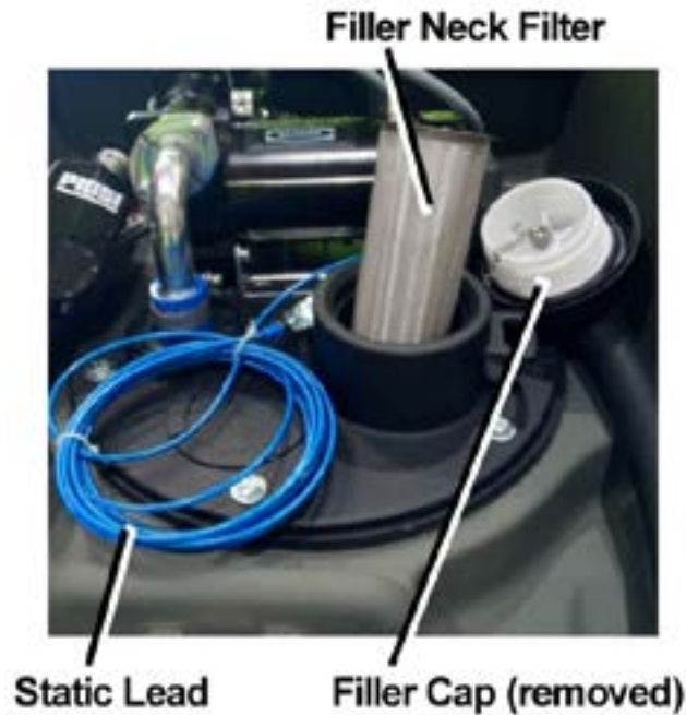
Figure 2 – Tank Filling Operation
