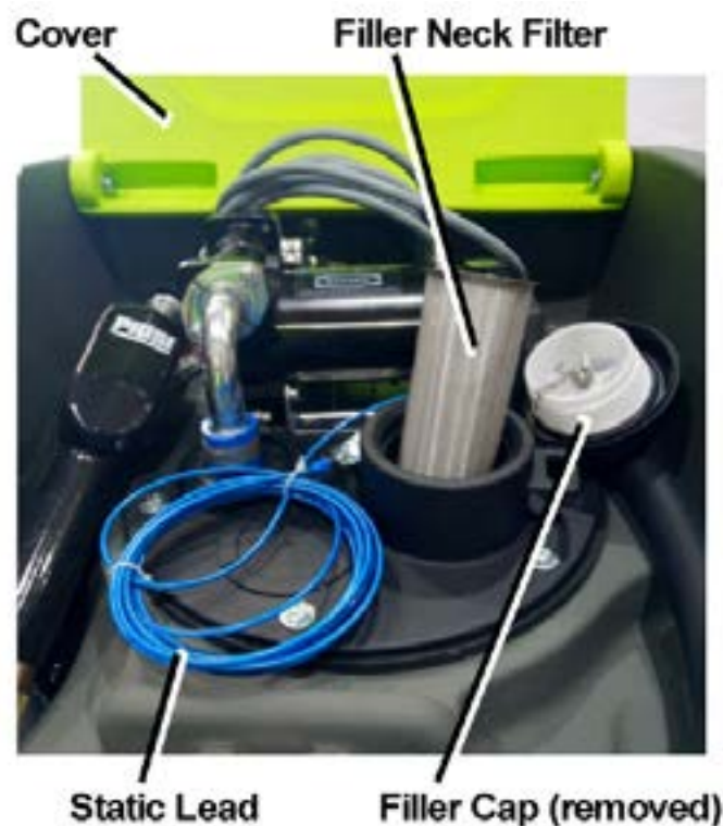
Figure 3 – Filling Operation
